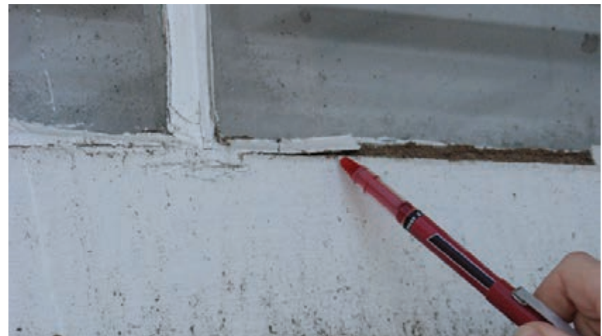
Figure 3.97 - Deteriorated window putty.
