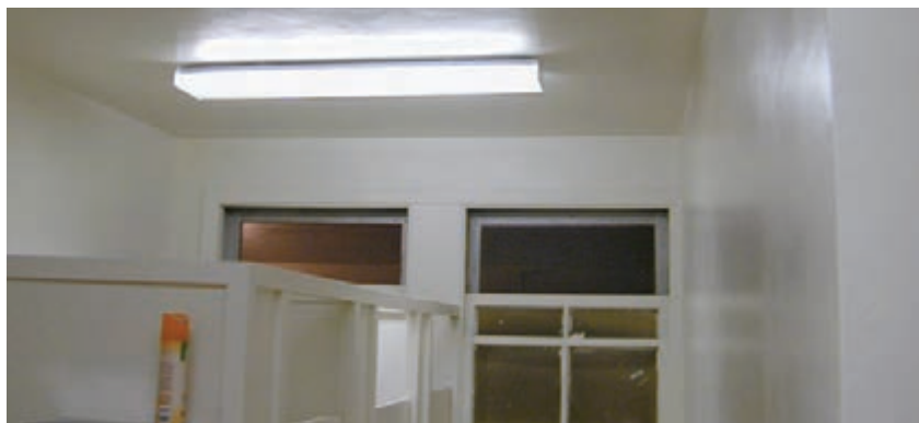
Figure 3.107 - Lack of exhaust fan in restroom and operable windows that no longer vent to the exterior.
