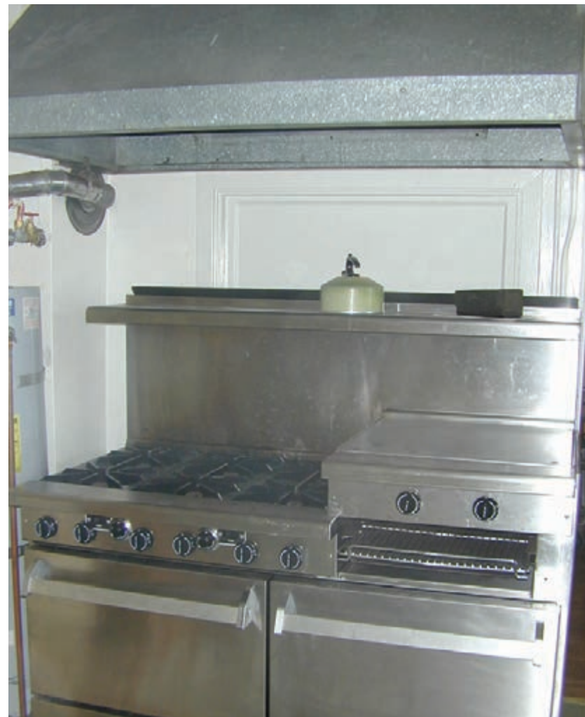
Figure 3.106 - Code deficient hood over kitchen range.
