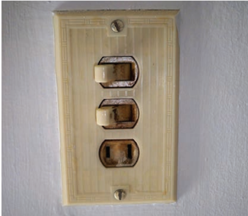
Figure 3.149 - Typical two-prong type receptacle.
