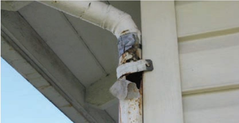
Figure 3.141 - Typical detachment at downspout connection.
