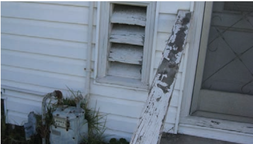
Figure 3.124 - Typical louvered vent at kitchen area.
