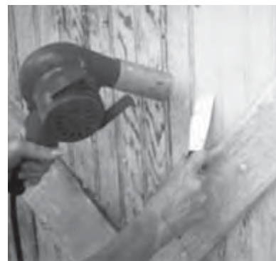
The nozzle on the electric heat gun permits hot air to be aimed into cavities on solid decorative
