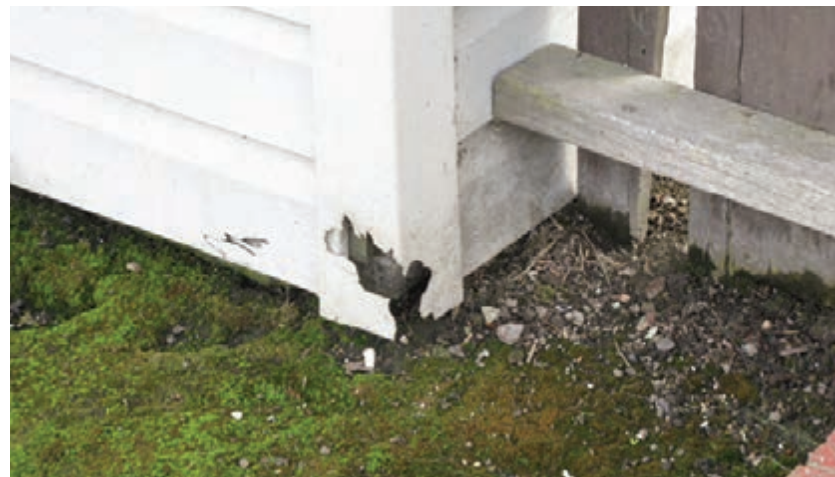
Figure 3.121 - Damaged vinyl siding.
