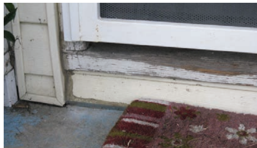
Figure 3.129 - Deteriorated wood threshold at door.
