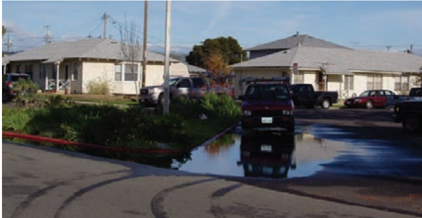
Figure 3.5 - Typical ponding at off street parking areas.
