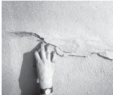
Applying a waterproof coating to an above-ground masonry wall can trap moisture underneath, causing further damage to the historic material. Photo: NPS files.
