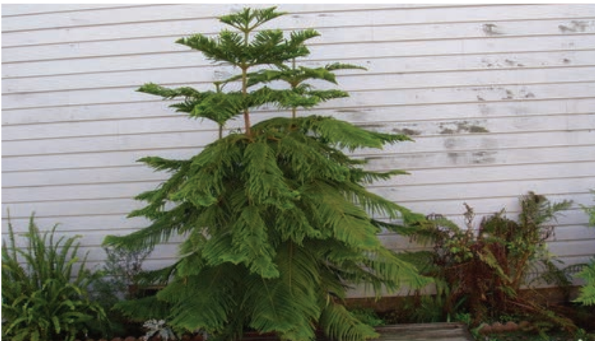
Figure 3.13 - Tree plantings located too close to the building foundation.
