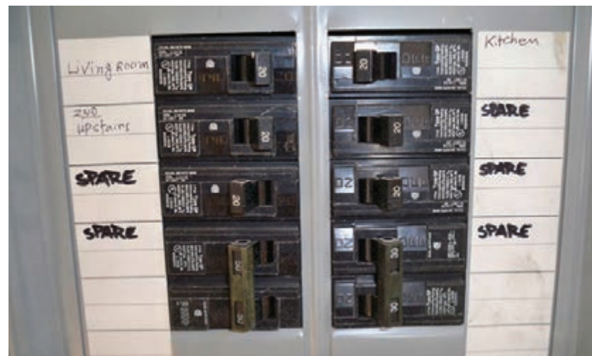
Figure 3.147 - Typical electrical panel
