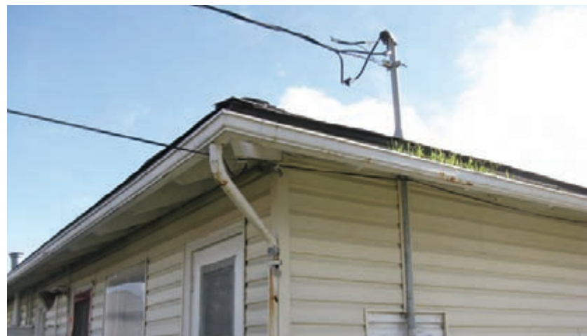
Figure 3.140 - Typical deteriorated gutter in need of maintenance.
