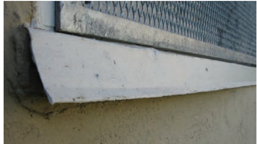
Figure 3.96 - Window with install flashing drip edge.
