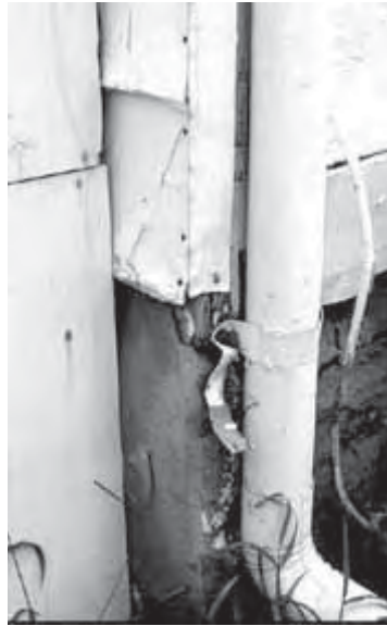
A clogged or broken downspout causes the water to pour directly into the ground. NPS files. Photo: NPS files.
