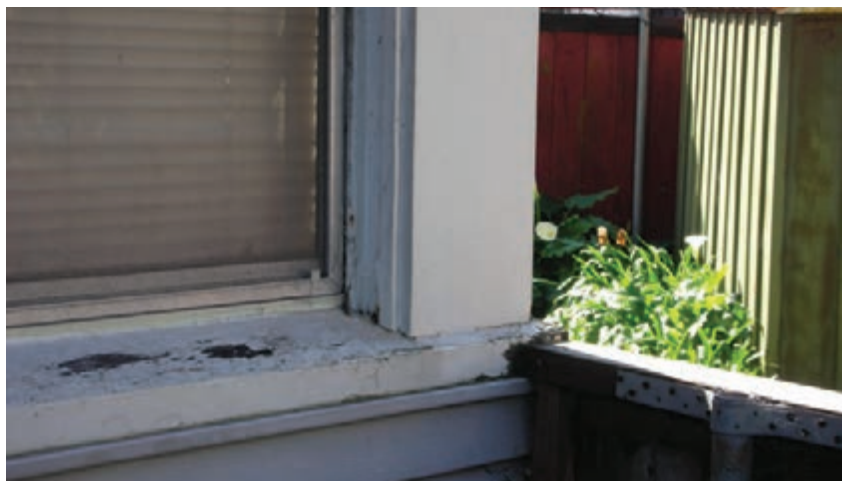
Figure 3.131 - Typical deterioration of wood sill and frame.
