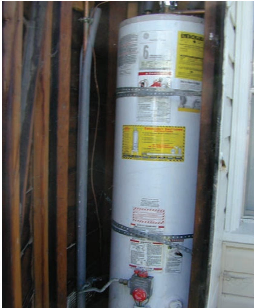
Figure 3.144 - Typical water heater located within storage blister at exterior.
