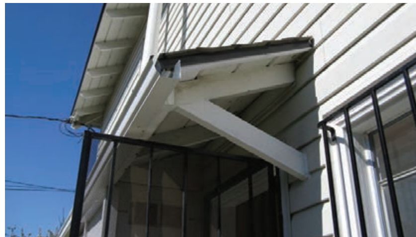
Figure 3.139 - Typical replacement aluminum gutter at main entrance.
