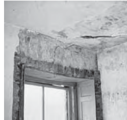
Damp interior plaster around windows generally indicates moisture has entered from the outside. Photo: NPS files.
