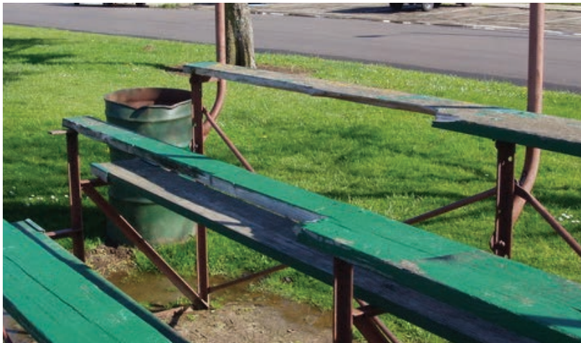
Figure 3.64 - Deteriorated bleachers at ball field.
