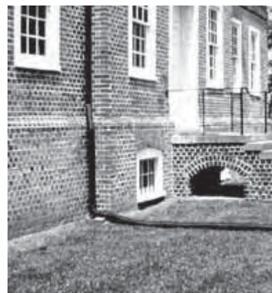
The owner used long black extender pipes to test a theory that it was faulty roof drainage causing the problem. Photo: NPS files.
