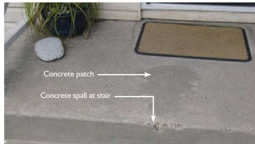
Figure 3.114 - Typical deterioration of concrete stair and landing.
