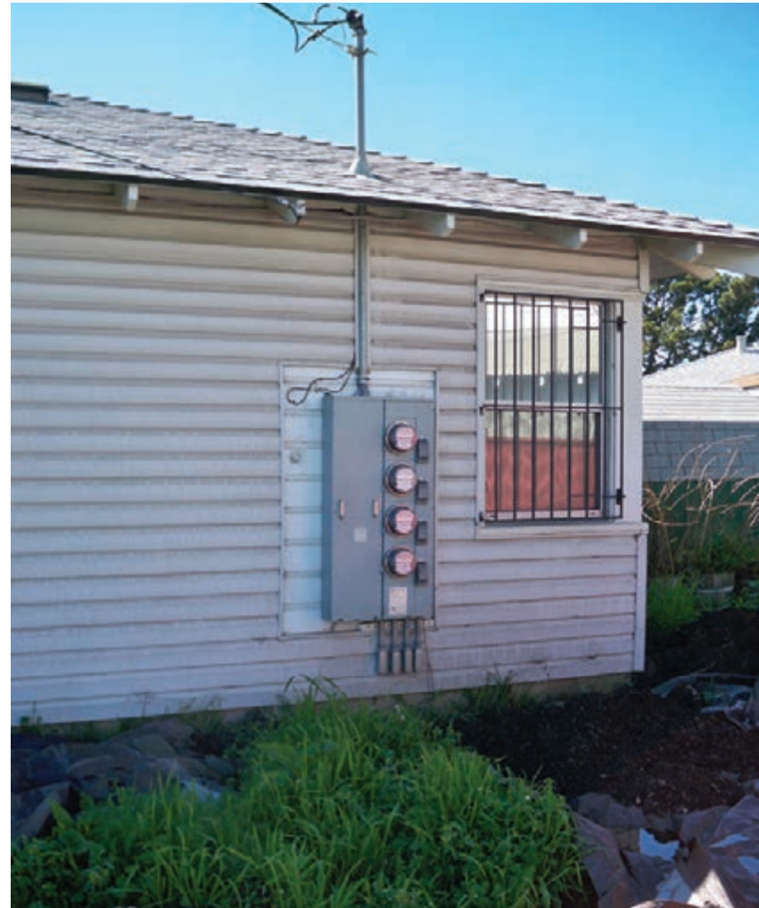
Figure 3.145 - Typical electrical service into unit.
