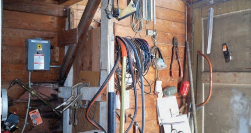
Figure 4.33 - Area where verification of electrical clearance is needed.
