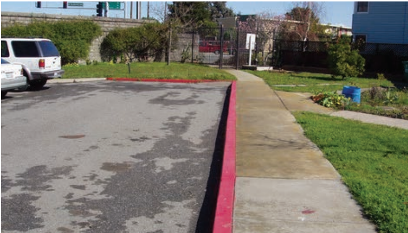
Figure 3.43 - Typical curb in good condition.
