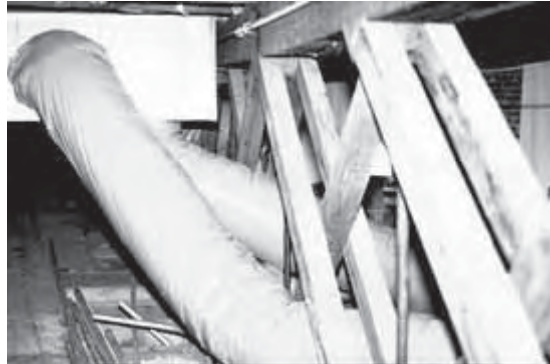
The flexible duct work, seen here, can be used to advantage in tight attic spaces. Photo: NPS files.
