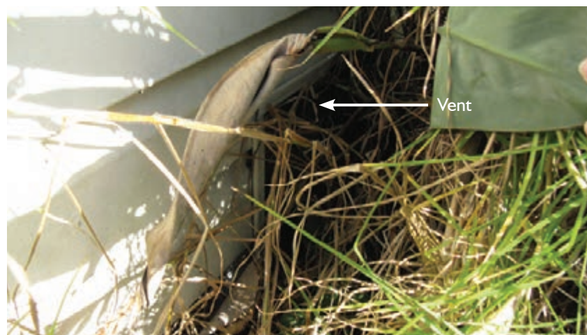
Figure 3.126 - Typical vent obstructed by plantings.
