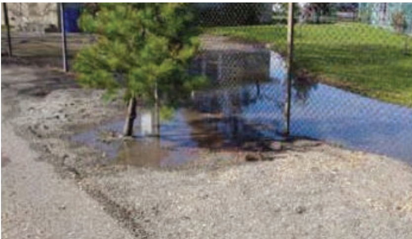
Figure 3.2 - Pea gravel used to raise grade in areas of flooding.
