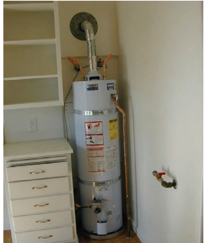
Figure 3.143 - Typical water heater within unit.
