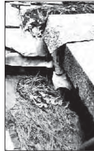
Debris will impede the normal flow of water from the roof's gutter and downspout system to the ground and result in moisture problems. Photo: NPS files.
