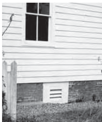
A vent may be added if there is none. Close grilles in the summer, if hot humid air is getting into air conditioned spaces. Photo: NPS files.
