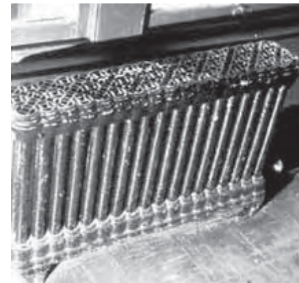
This radiator would be identified as a significant element of the interior. In any work to upgrade the mechanical system, it would be retained and preserved, even if non-functioning. Photo: NPS files.
