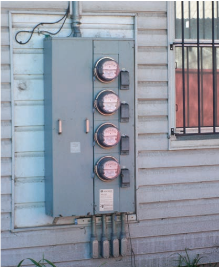
Figure 3.146 - Typical meter and main circuit breaker.
