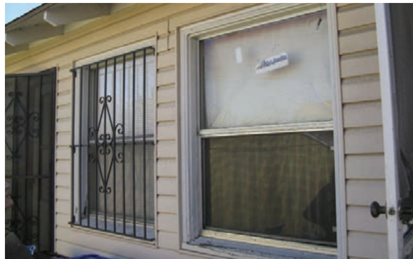
Figure 3.132 - Typical aluminum sash replacement window and security grill.
