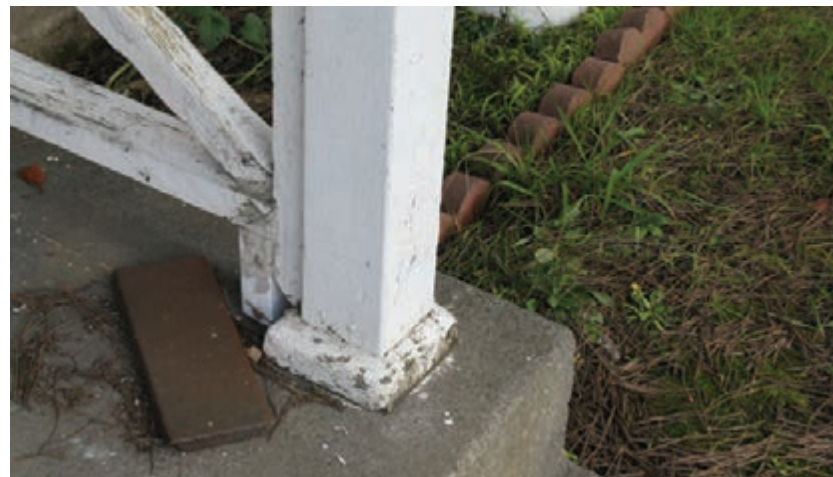
Figure 3.117 - Deterioration of porch column due to paint failure.
