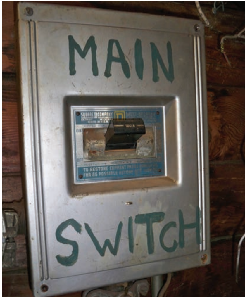
Figure 3.109 - Main circuit breaker.
