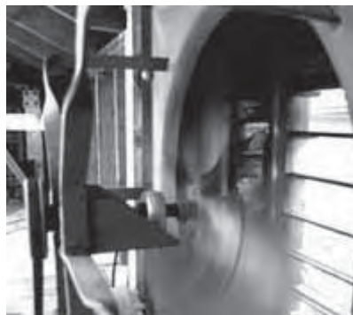
Installing ventilating fans can improve damp conditions or reduce cooling loads. Photo: NPS files.
