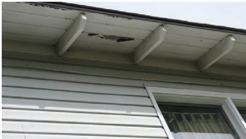
Figure 3.137- Typical paint failure at underside of soffit.
