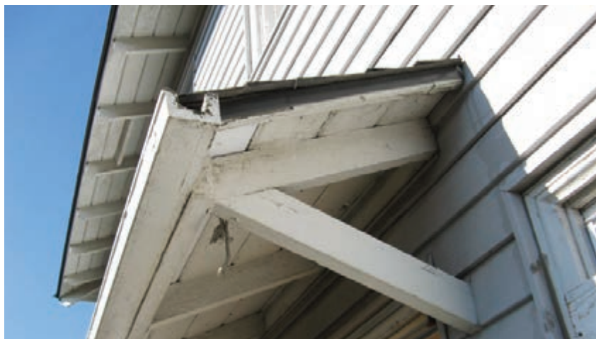
Figure 3.138 - Typical historic wood gutter at rear entrance.
