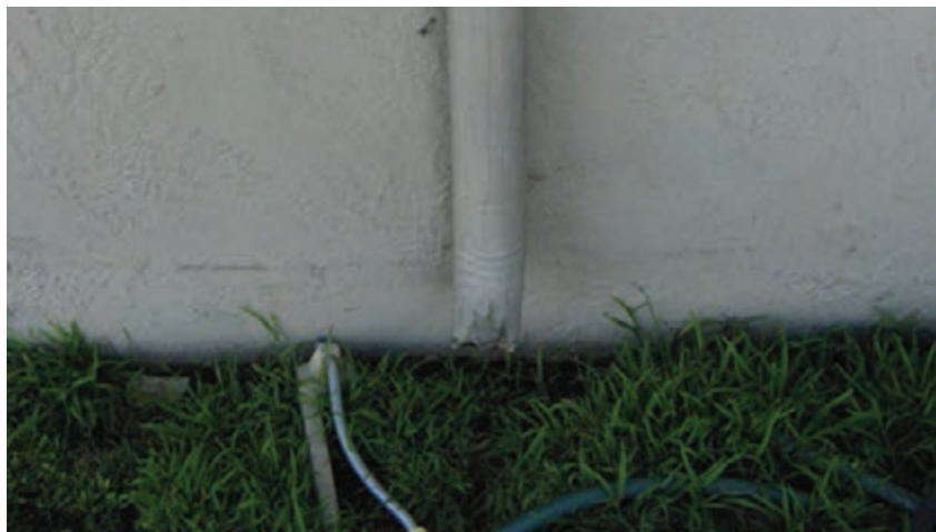
Figure 3.101 - Downspout without splash pad to direct water away from foundation.
