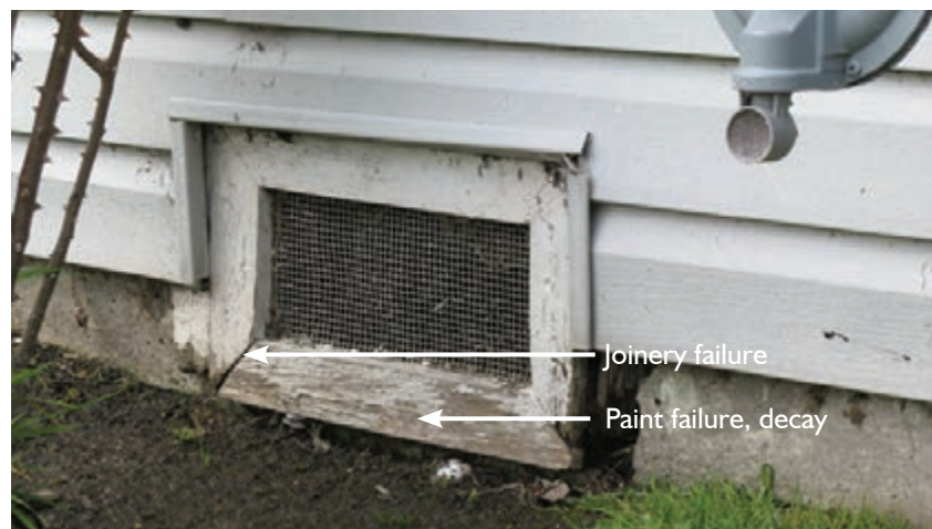
Figure 3.125 - Typical deteriorated wood sash vent.
