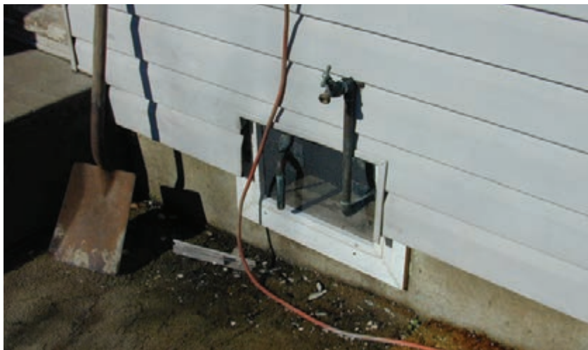
Figure 3.153 - Typical hose bib and water service.
