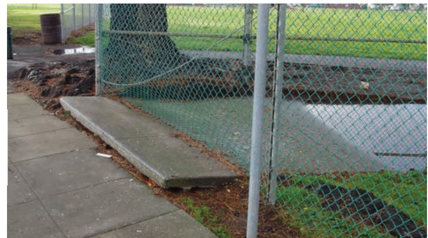
Figure 3.42 - Sidewalk damage due to tree root system.
