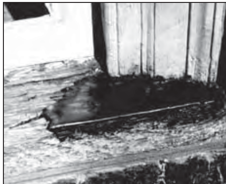
This illustrates a two-part epoxy patching compound used to fill the
