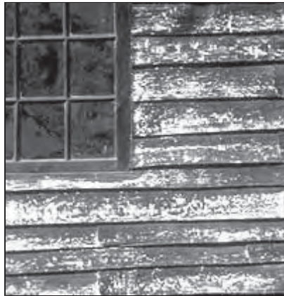
Historic wood siding exhibits rich and varied surface textures. They range from hand-split clapboards of short lengths with feather-edged ends (shown here), to pit or mill sawn boards which can be beveled, rabbeted, or beaded. Photo: NPS files.
