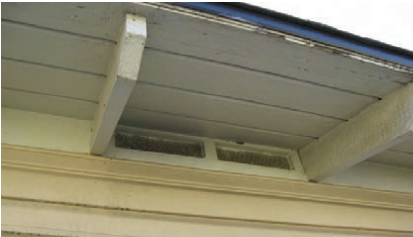
Figure 3.136 - Typical attic vent.
