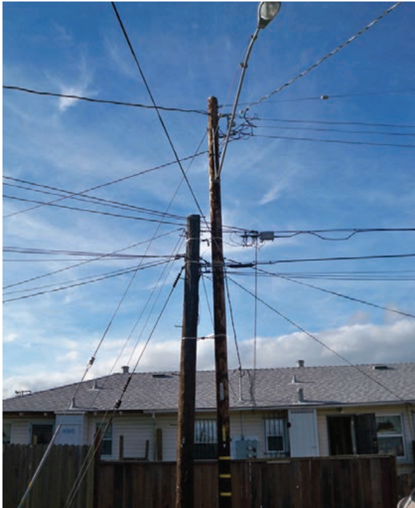
Figure 3.108 - Typical overhead electrical service.
