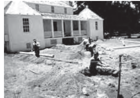
New drainage systems for roof run-off may be installed in order to remove moisture from the base of the building. Photo: NPS files.
