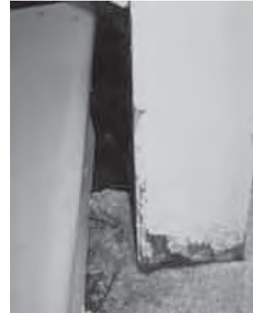
The problem evidenced here by mossy growth and deteriorated wood must be resolved and the wood allowed to dry out before the wood is repainted. Photo: NPS files.
