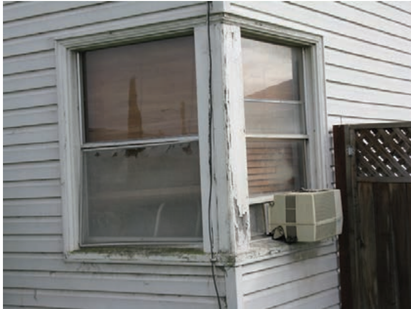
Figure 3.133 - Typical corner window in poor condition.
