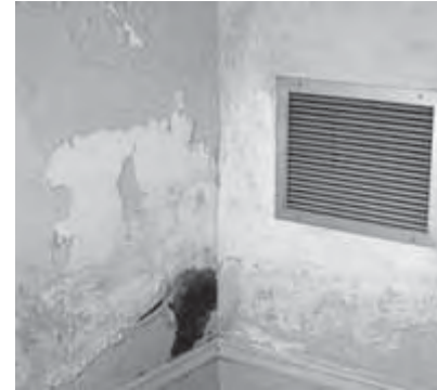
If adequate ventilation is installed, damage to interior walls such as this can be prevented. NPS files. Photo: NPS files.
