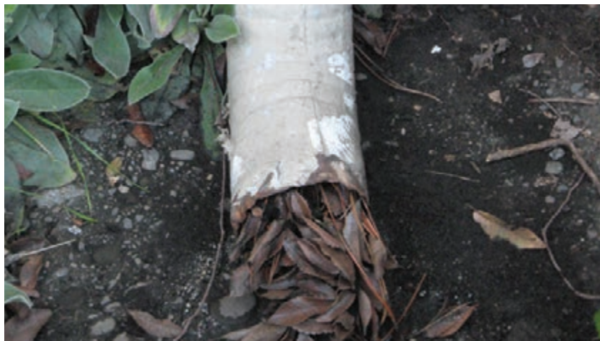
Figure 3.100 - Typical clogged downspout.
