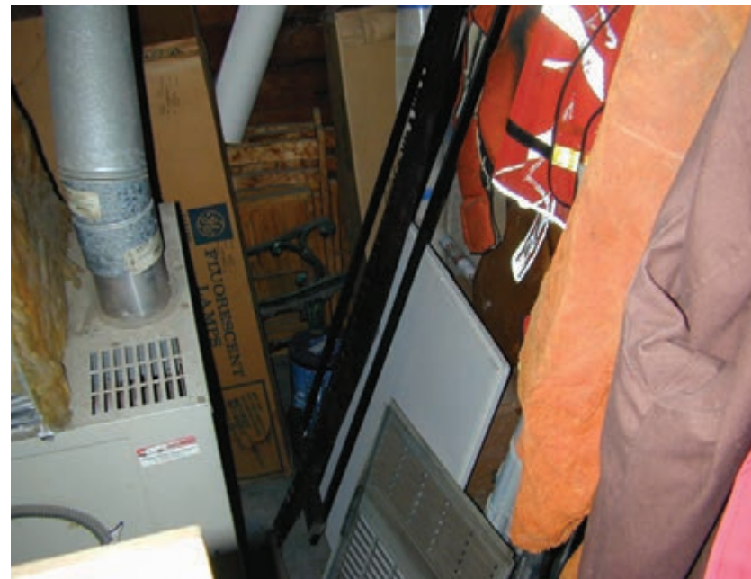
Figure 3.104 - Lack of clearance at path of travel in front of furnace.
