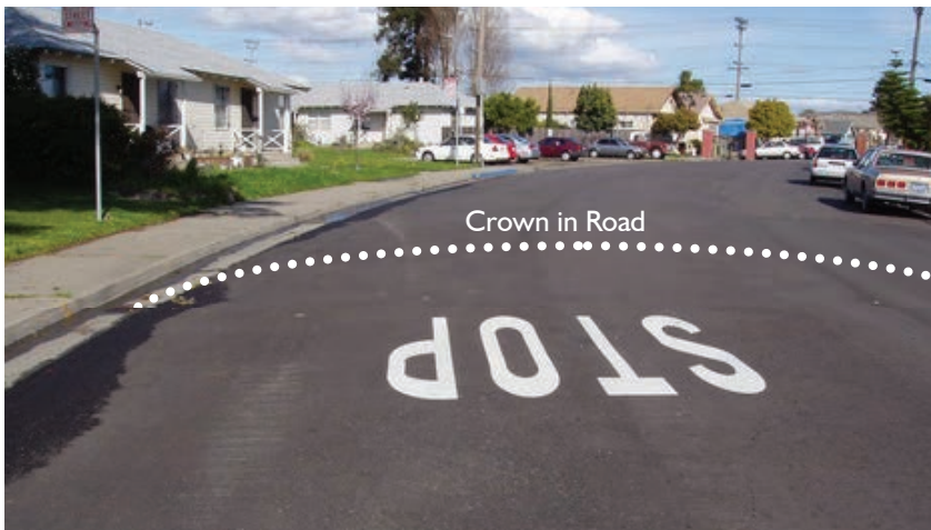
Figure 3.40 - Typical crown in road.
