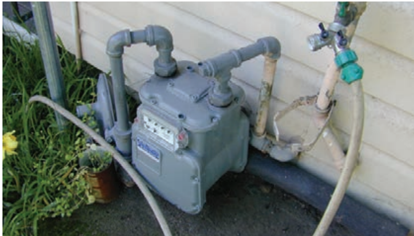
Figure 3.152 - Typical gas meter.
