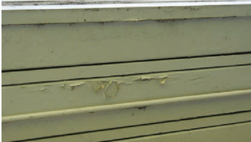
Figure 3.98 - Typical soffit showing paint deterioration.
