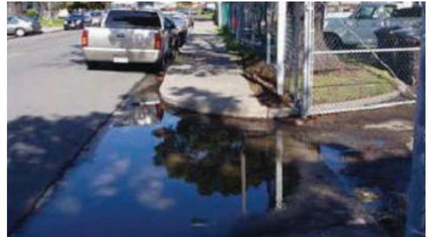
Figure 3.3 - Typical water ponding at curb cuts.
