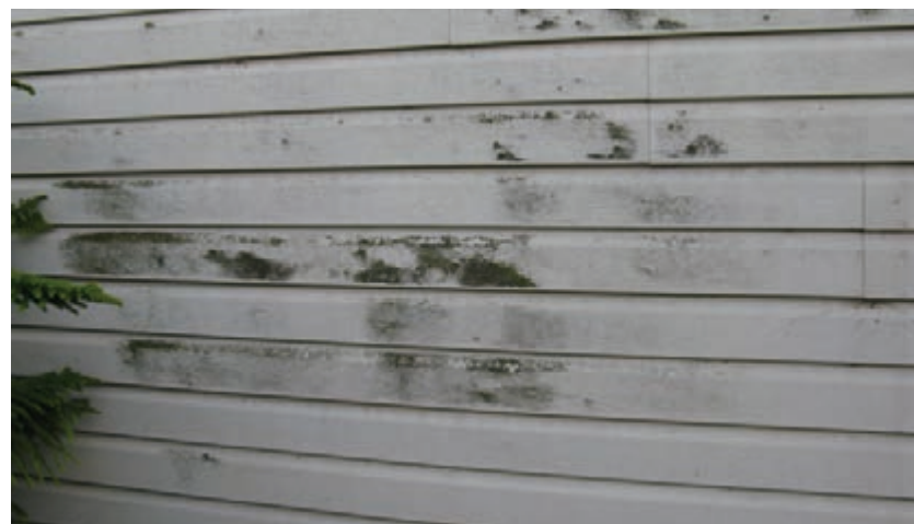
Figure 3.122 - Organic growth on vinyl siding.
