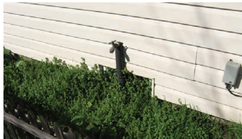
Figure 3.127 - Typical vent obstructed by planting bed.
