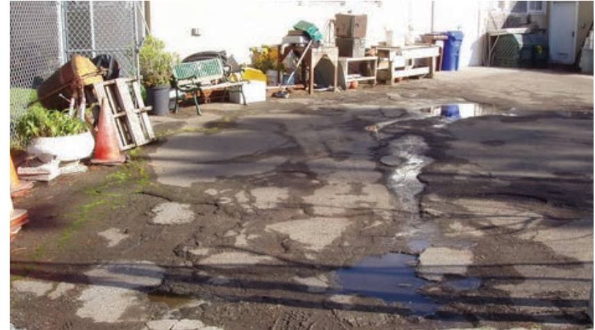
Figure 3.41 - Service yard paving in poor condition.
