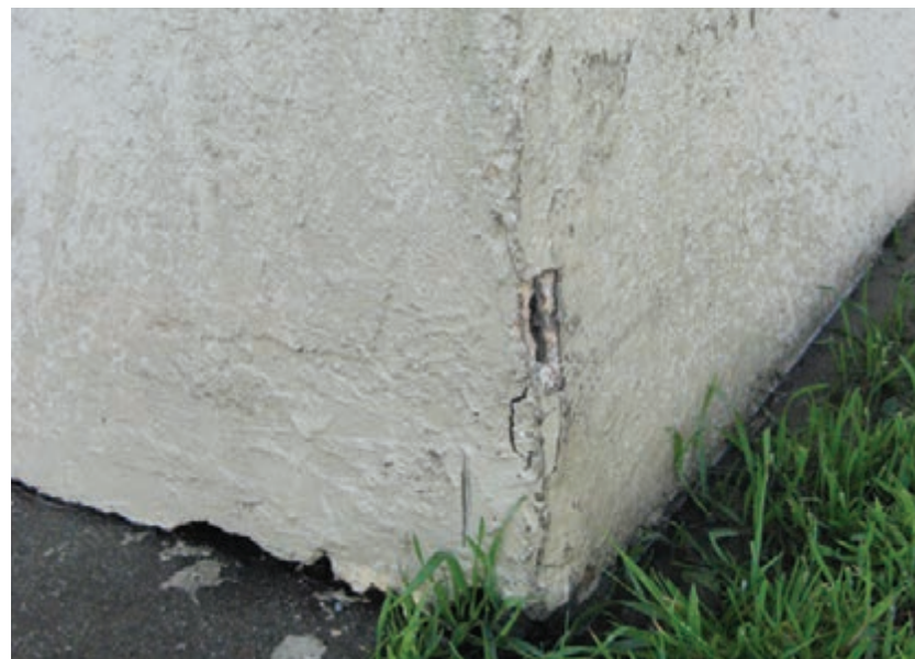
Figure 3.87 - Deteriorated stucco at building corner.
